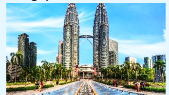
Petronas Twin Towers
